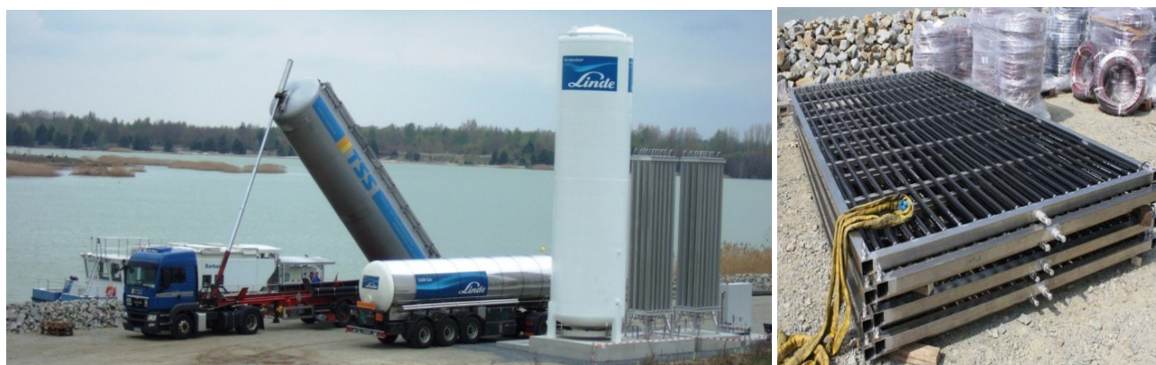
Fig. 17: At left: Vertical tank being filled with liquefied CO 2 , and the water treatment vessel (behind lorry) being loaded with calcium hydroxide; and right: gas delivery frame with micro pores before installation on the lake bed (source: LMBV)
