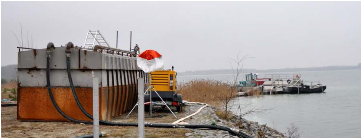
Fig. 9: Pre-mixing container and Puma water treatment vessel using the submerged turbulent-jet input technique (source: BGD)
